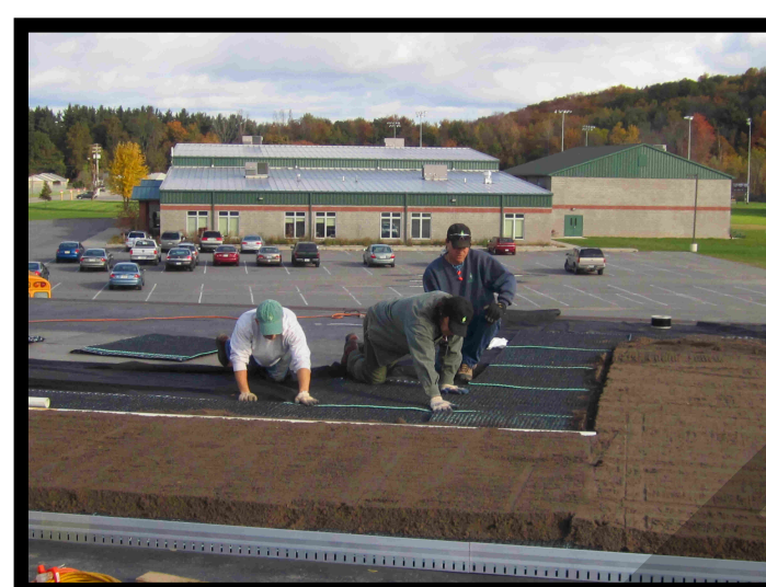
Screed Growing Media to Spec *DO NOT Exceed Loading
