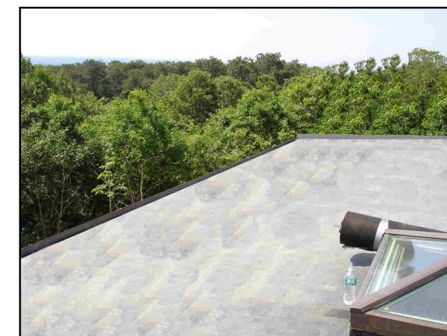
Clean Roof Deck
