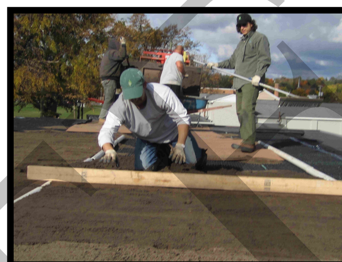
Screed Growing Media to Spec *DO NOT Exceed Loading
